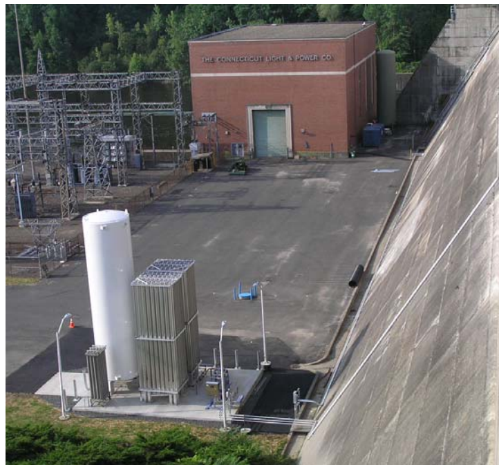
Figure 1: Shepaug Dam Powerhouse and Oxygen Supply Facility
