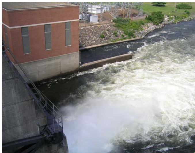
Figure 3: Spilling Procedures at Shepaug Dam
