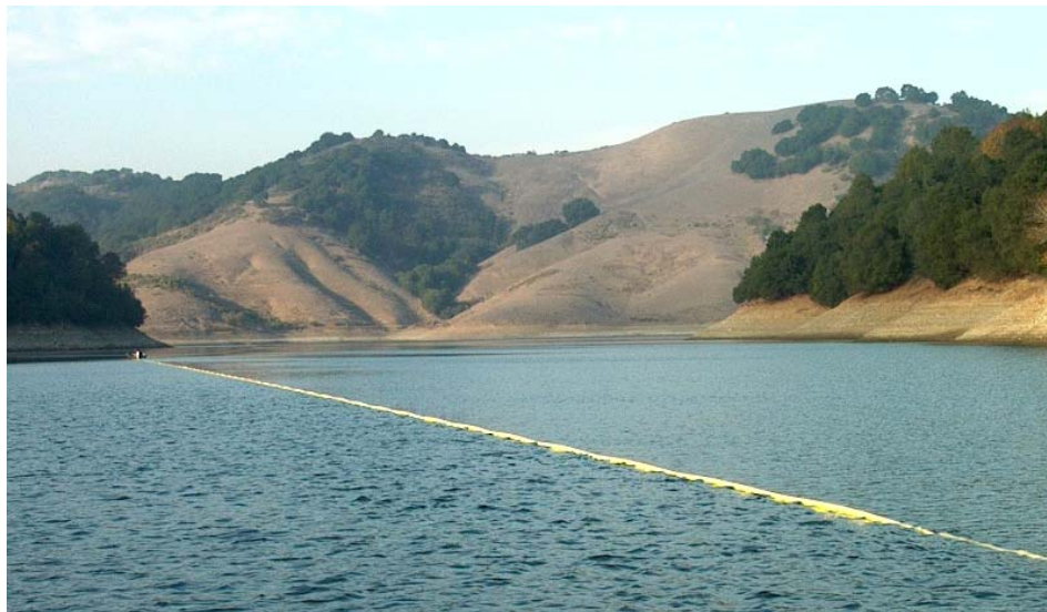
USL Diffuser Prepared for Deployment
